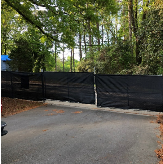
Wind Screen Installed at Site Entrance
